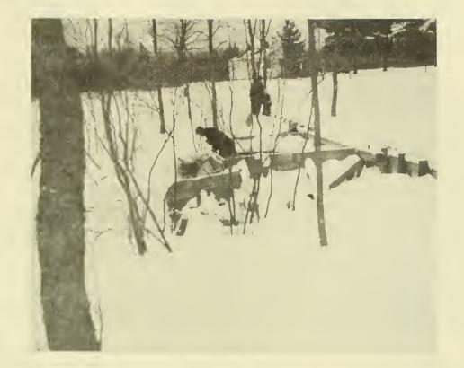
Figure 60.--Carp Lake River dam and inclined-screen-trap in operation during winter months. Trap box has been removed and replaced by a baffle across the foot of the inclined screen. February, 1949.
